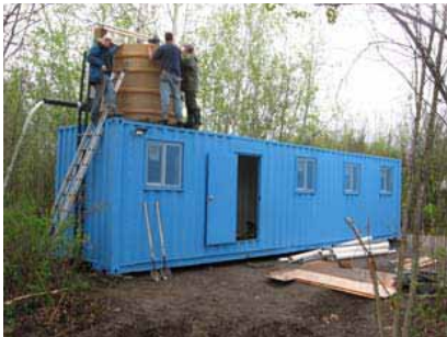
2006 Vanderhoof Pilot Facility
