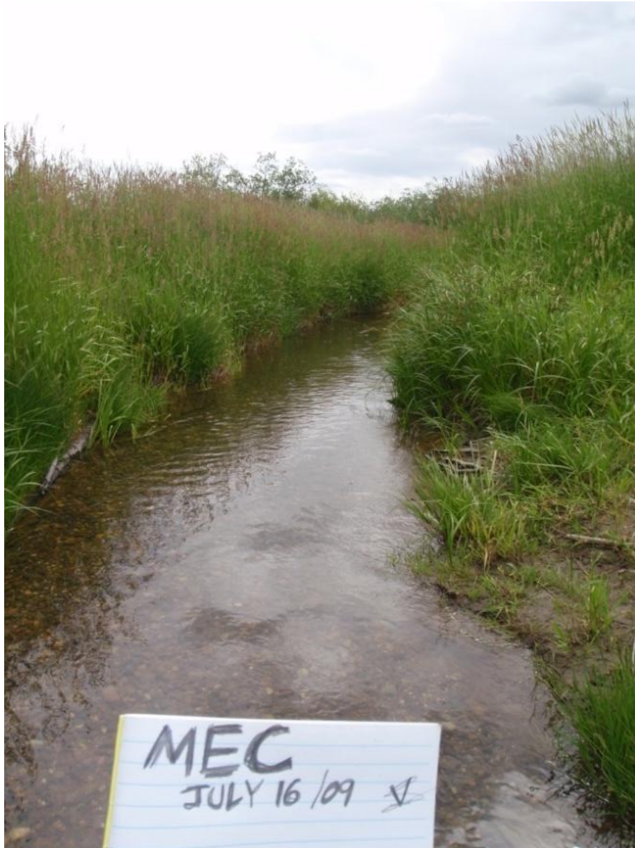
Plate 1: Gravel placed into upstream section of Site 2, July 16, 2009.
