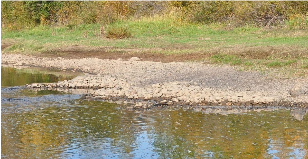
Photo 9: Placed substrate that is emerged out of the water is visible near the river bank while native gravels can be seen along the edge of the river bank. Photo from Lower Patch on left bank.
