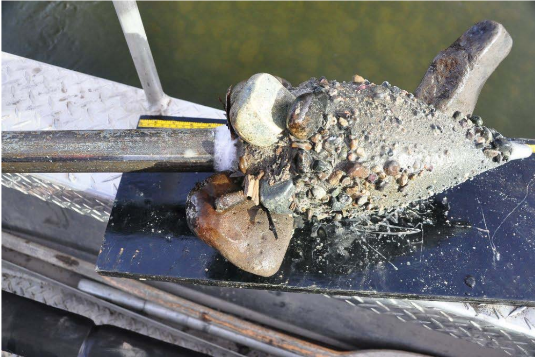
Photo 63: Core 18 (Lower Patch)
