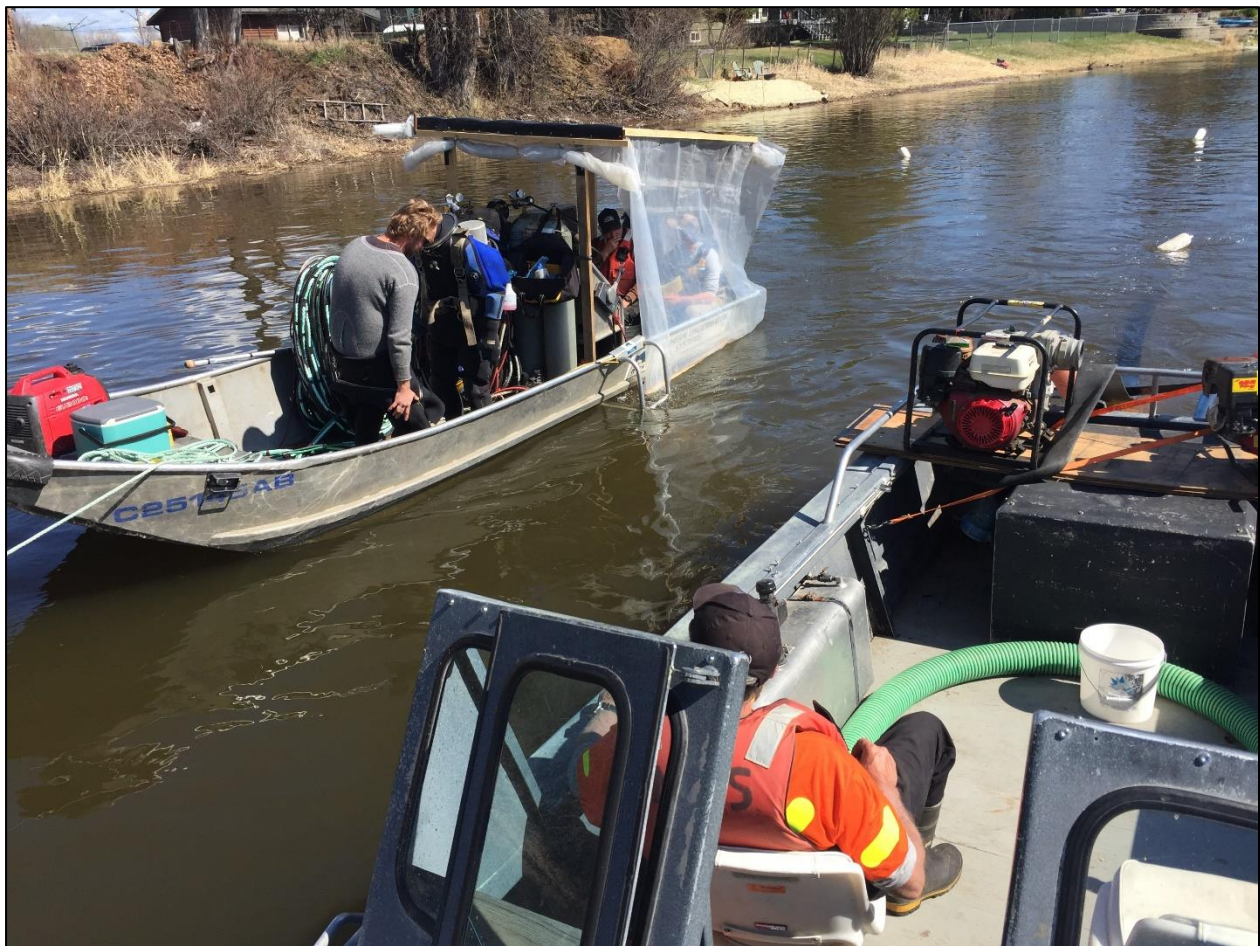
Photo 2.1 Divers preparing to perform substrate cleaning at Lower Site on May 7, 2020; note area to be cleaned marked by white buoys, as well as the slurry discharge line used to relocate dredged sediment (black hose trailing downstream).
