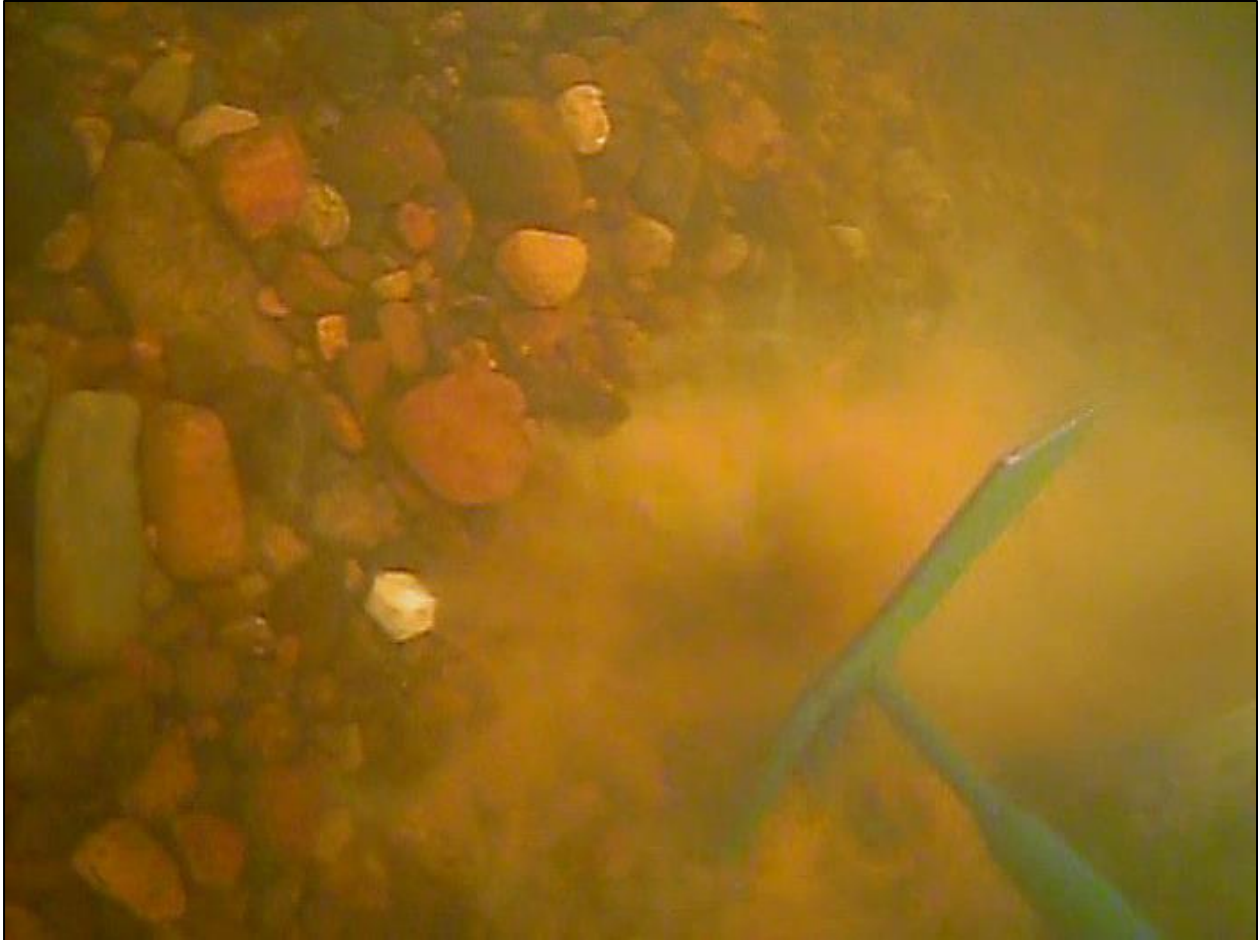
Photo 2.3 Mechanical raking used in combination with the suction dredge to remove infilled fines from the subsurface layers (flow left to right; substrate at top-left of image has been cleaned).
