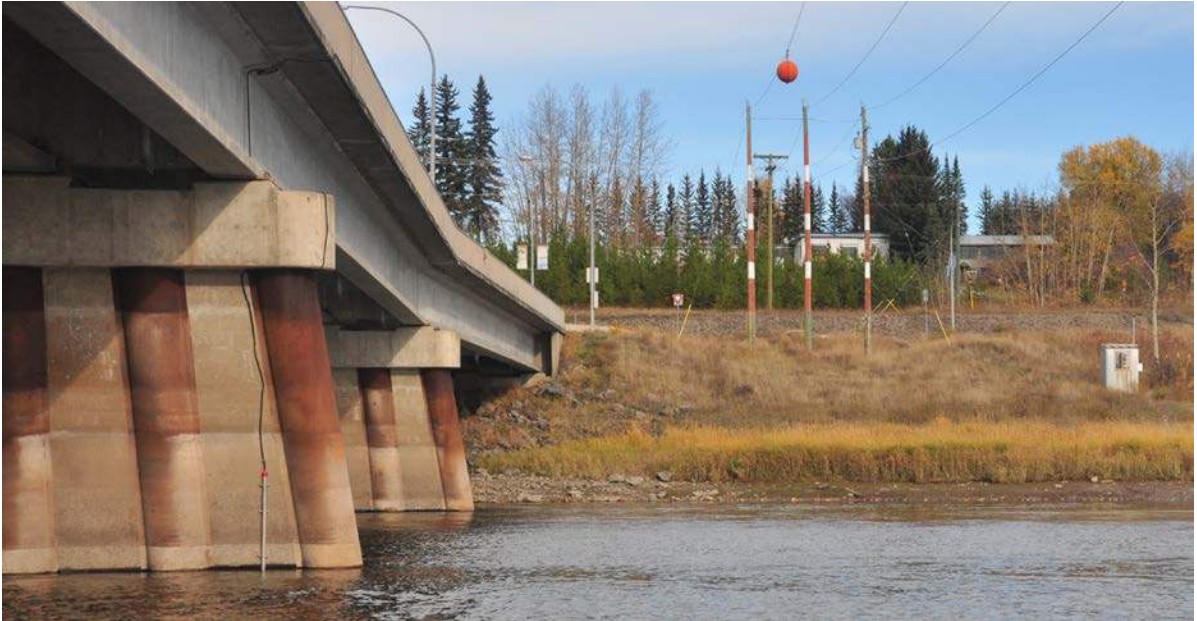
Figure 13 Turbidity sensor installed on middle pier of Burrard Avenue Bridge.
